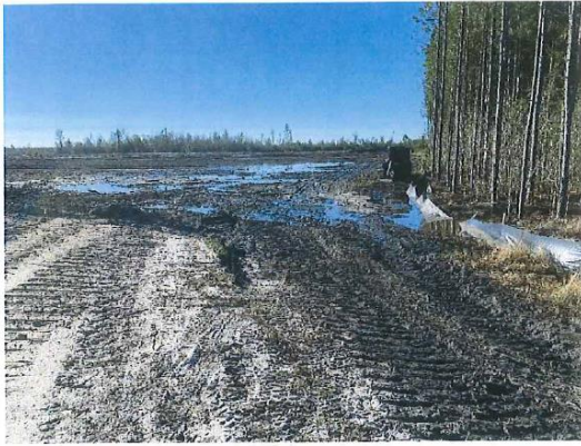
Area 2 Water on Topsoil return area (January 31, 2024)
