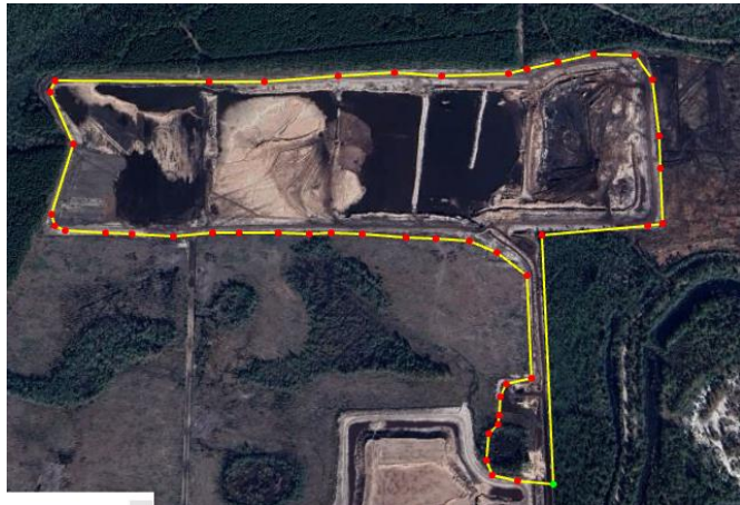
Location 1 Northwest Mine Cell
