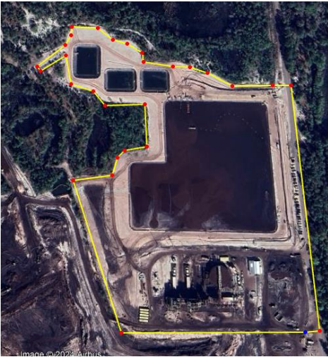
Location 3 IWW Treatment Ponds, Process Pond, and Plant Units
