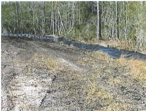
Silt Fence Repaired (January 31, 2024)
