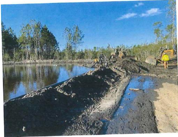
Northwest corner Reclamation cell (January 31, 2024)
